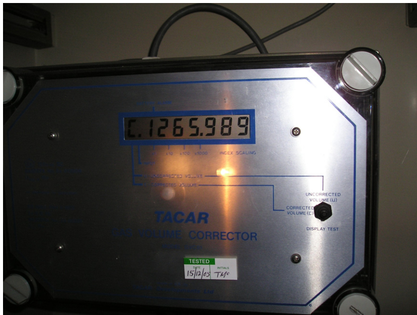
Fig. 1. The interface of the gas corrector meter in the input pipe to Edinburgh University's central area combined heat and power plant. Photograph courtesy David Somervell, Estates and Buildings, University of Edinburgh.
